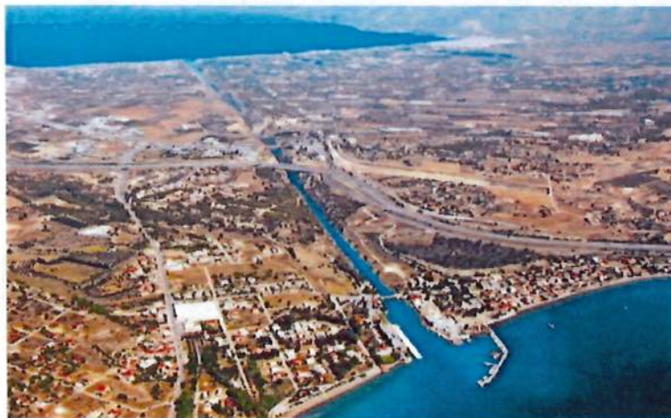
Corinth Canal (Source: Google Images)
