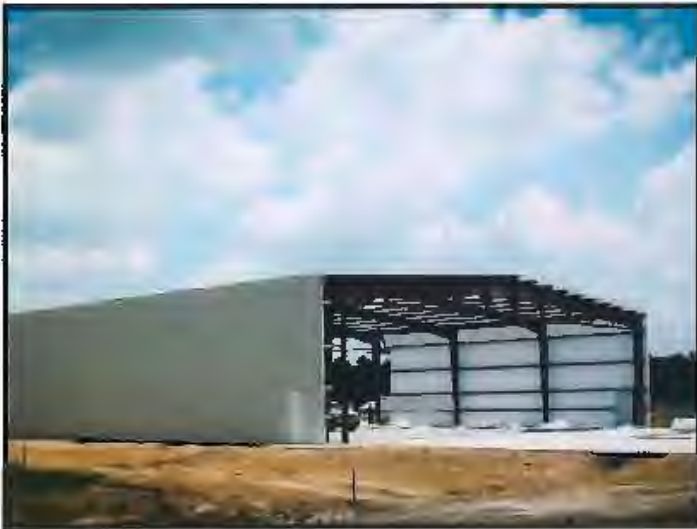
Numerous other Airplane Hangars—All Pre-Engineered Metal Buildings Sizes Ranged from 80'x80' up to 100'x150' and up to 28' Eave Heights
