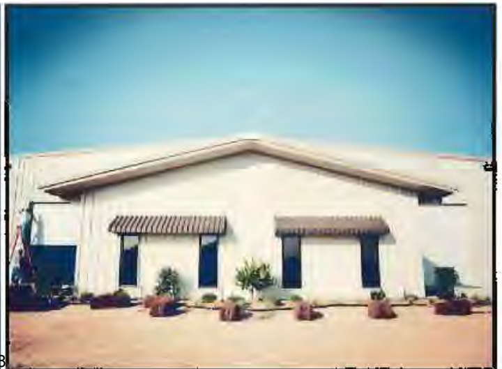
Numerous other Airplane Hangars—All Pre-Engineered Metal Buildings Sizes Ranged from 80'x80' up to 100'x150' and up to 28' Eave Heights
