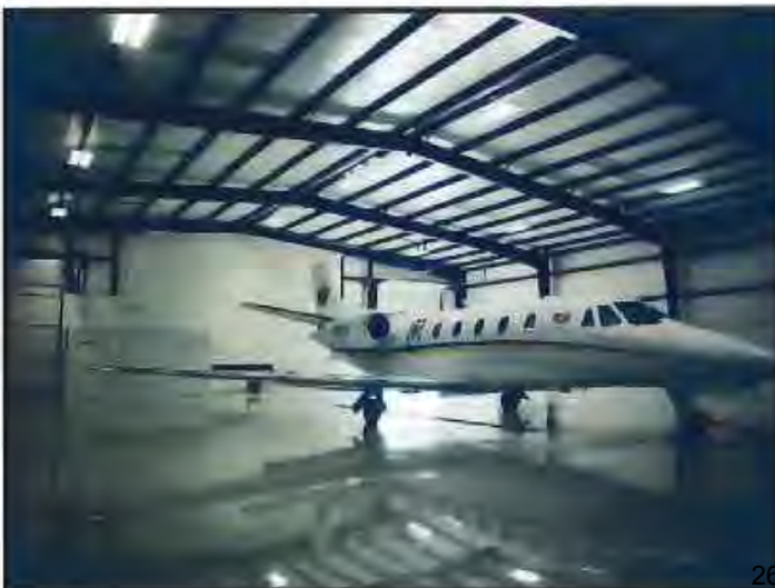
Numerous other Airplane Hangars—All Pre-Engineered Metal Buildings Sizes Ranged from 80'x80' up to 100'x150' and up to 28' Eave Heights
